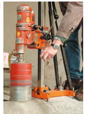
2. Wet the whole bored surface, if dry, with a good amount of water. Allow the water to be absorbed by the bored surface, until all water drops are gone\*.
