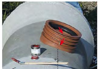
4. Before the mounting of the connection pipe **DS BAST GV** has to be applied on the sealing ring in the socket of the connector and on the pipe spigot end. In case of a cut pipe its end has to be bevelled before.
