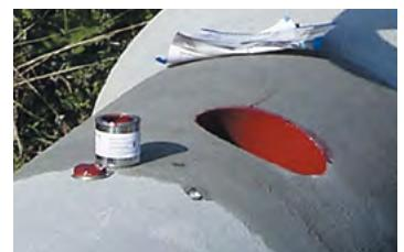
3. Press the pipe connector centrally – with its mark in axial direction of the pipe – into the bored hole until the stop is reached. Centrical insertion is important, in order to compress the first rubber rib evenly and to avoid its turn over.
