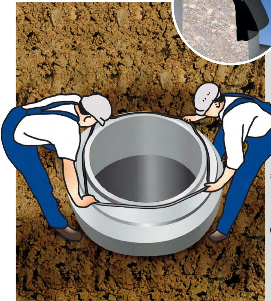
1. Pull seal on the cleaned spigot end, with the slide mantle showing upwards and to the outside.
